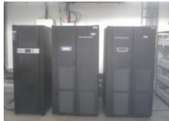
Disconnection of 2x80KVA & 2X20 KVA UPS's
